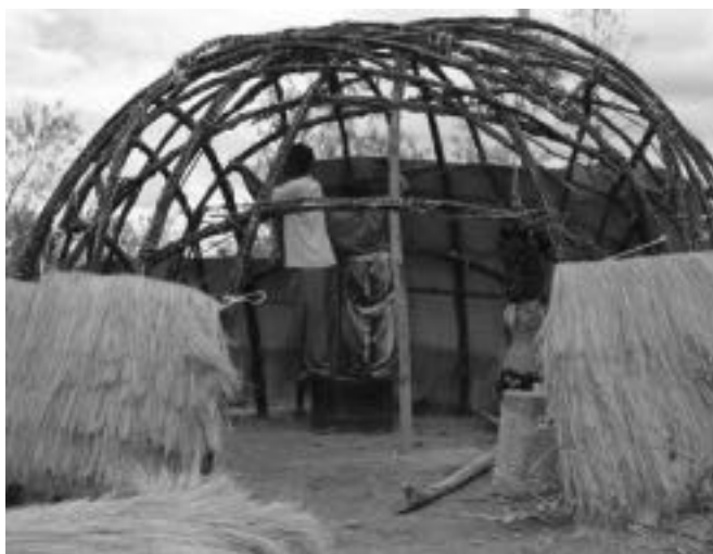
Figure 7.5. Sisal-thatch cover.
